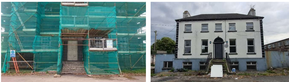
Fig.30: Protective wrapping to scaffolding at Dowth Hall (L), Front façade of Glebe house (R)
