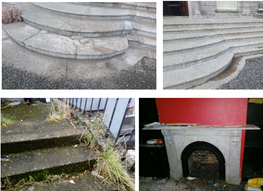
Fig.35: Before (TL) and After (TR) images of step repair at Charleville House. (BL) Existing external steps at Glebe House; (BR) existing marble fire piece at Glebe House
