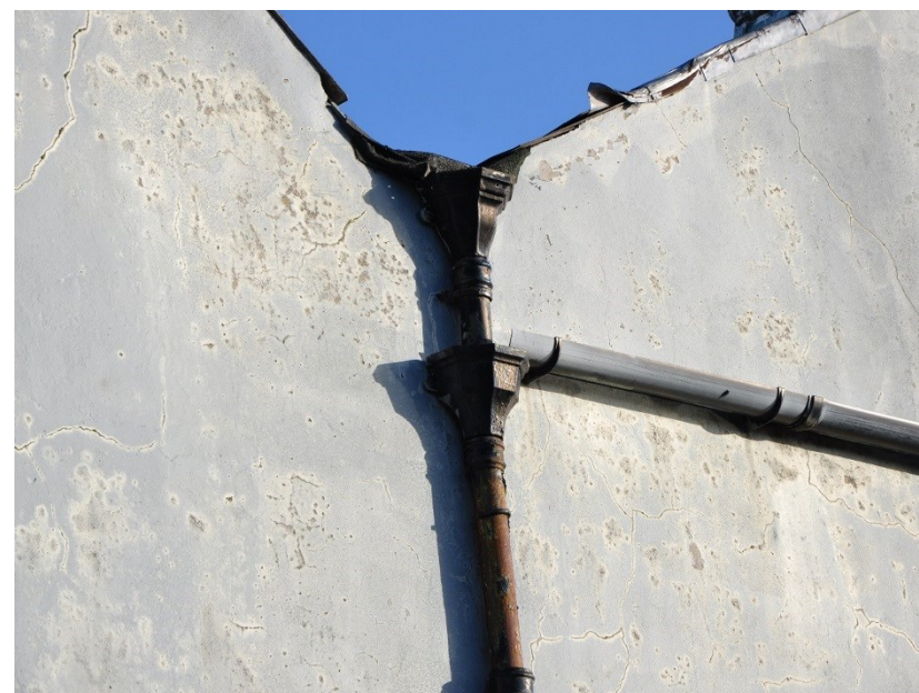
Plate 16: Detail of downspout/leader and two leader heads
